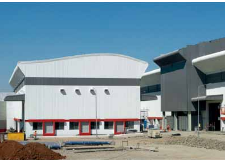
Dedicated testing facility for high pressure pumps
