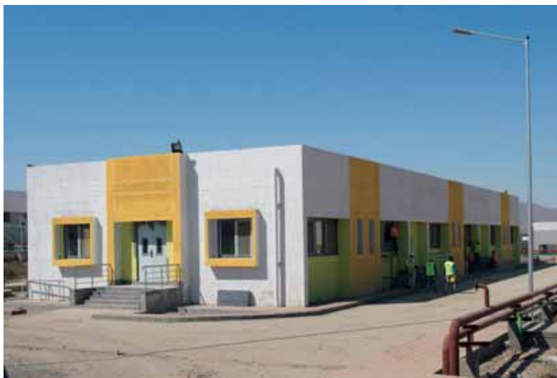
Canteen facility for employees
