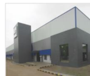
Foundry Division, Vambori
