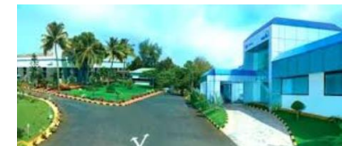
KSB MIL Controls Ltd. Meladoor, Kerela
