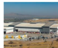
Energy Pumps Division, Shirwal
