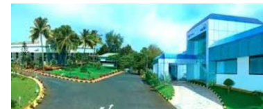
KSB MIL Controls Ltd. Meladoor, Kerela
