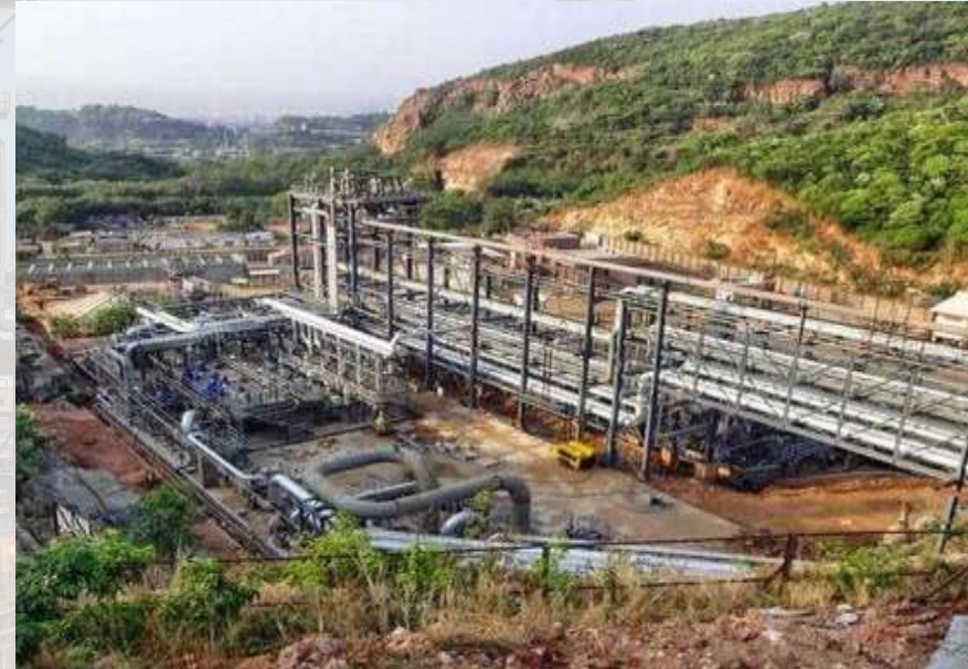
LPG cavern reference project, India
