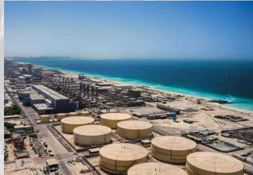
South Korea Doosan Yanbu IWP plant – € 1.2 million – butterfly valves
