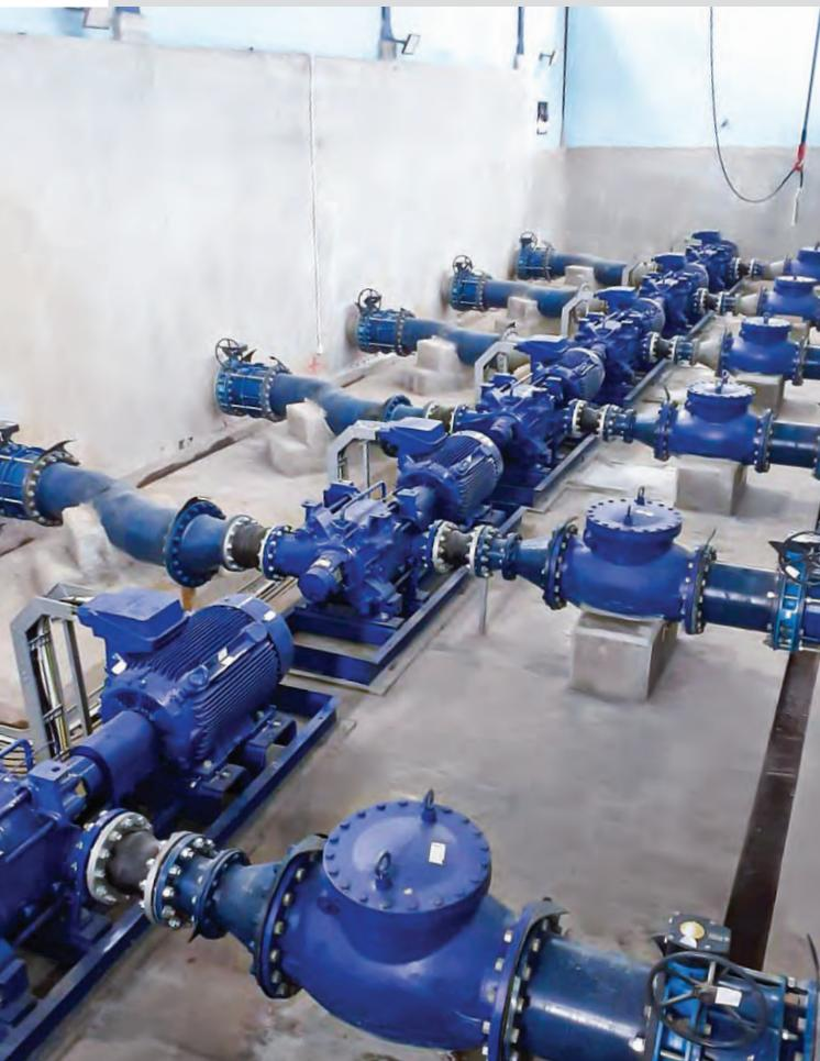
The SPAM in Bandar Lampung has been inaugurated in November, 2020. KSB Indonesia is proud to support this project by supplying a total of 25 units of 5 units of Sewatec (capacity: 210 lps, head: 25 m), 6 units of Multitec (capacity: 150 lps, head: 127 m), 5 units of ETN (capacity: 18.05 lps, head: 40 m), 5 units of Etanorm (capacity: 77.22 lps, head: 10 m), and 4 units of KRTK (capacity: 8.47 lps, head: 13 m).
